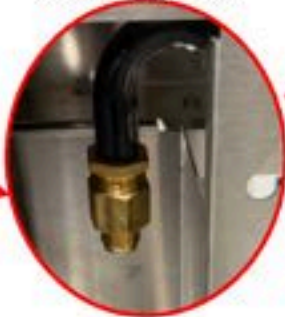
Fig. 2 Gas Connection
