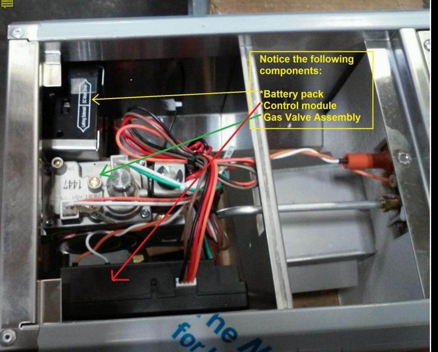
\*To remove the battery pack you'll need to gently press down on the battery pack to release it from the holder.
